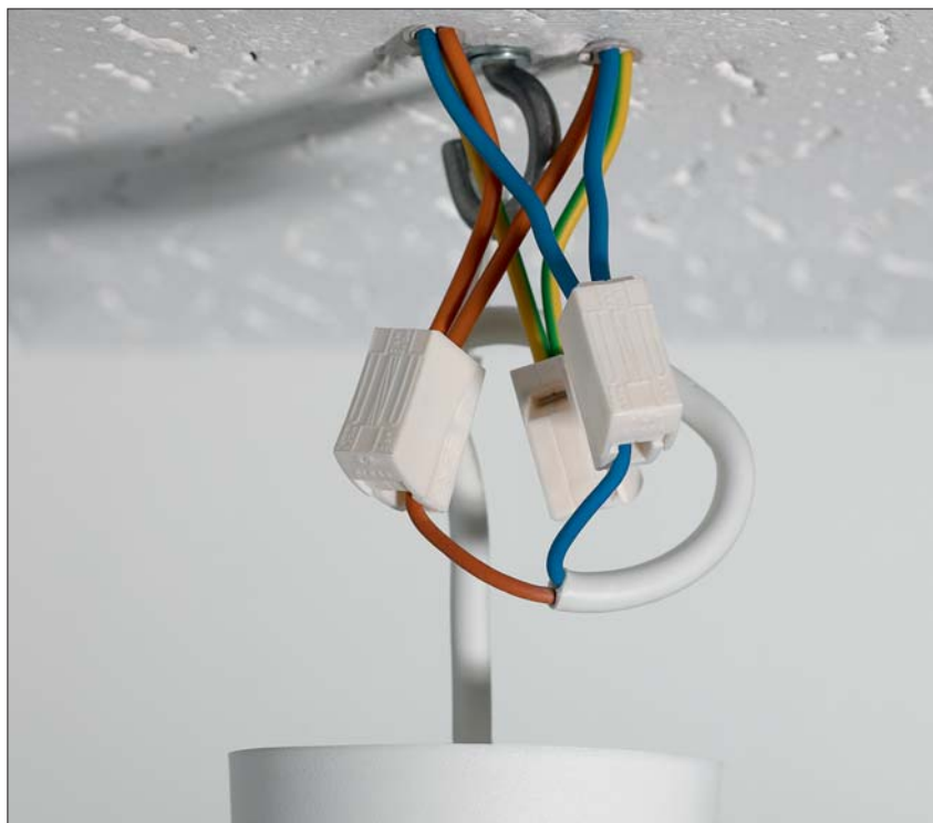
Quick installation and release of lighting devices with HelaCon Lux.
